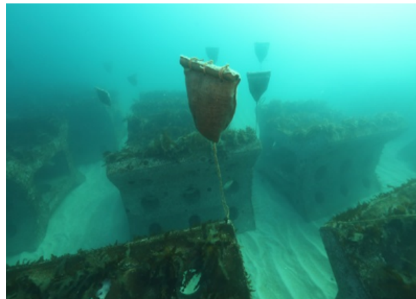
Restoration of kelp forests in Korea using concrete structures and seeding techniques. © FIRA
