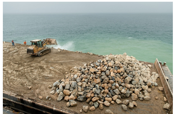
Barge deploying quarry boulders to create an artificial reef to recover a local giant kelp forest. Photo: San Clemente Times
